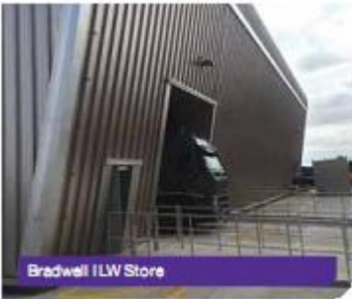
A DCIC itself incorporates a significant degree of shielding and as such a facility for its storage requires relatively little additional shielding and is simple in terms of construction.
