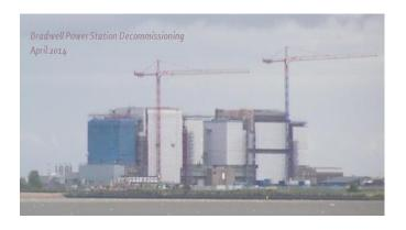
The main buildings at the UK's shuttered Bradwell nuclear power plant are being sealed in a £20 million (\$31 million) 'weather envelope' while they await final dismantling.
